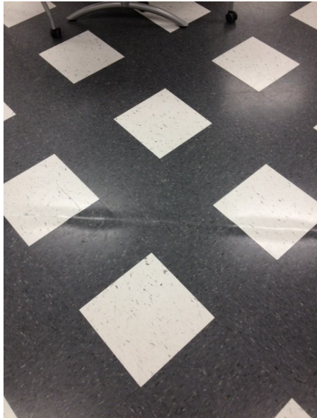
VCT Buckling over moving Expansion Joint
