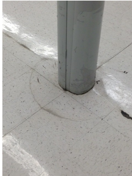
VCT Breaking around Support Column
