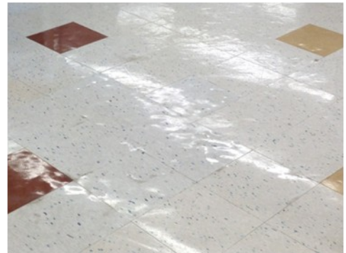
High spots in subfloor getting burned while burnishing Wavy & uneven subfloor telegraphing. Owner did not want to pay for prep, now he's complaining
