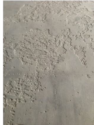
Poor concrete. Existing Tile was removed and did this to the subfloor. GC wanted flooring contractor to only skim the floor, not take care of the subfloor issue.
