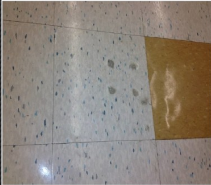
High spots in subfloor getting burned while burnishing Wavy & uneven subfloor telegraphing. Owner did not want to pay for prep, now he's complaining
