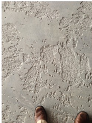
Poor concrete. Existing Tile was removed and did this to the subfloor. GC wanted flooring contractor to only skim the floor, not take care of the subfloor issue.
