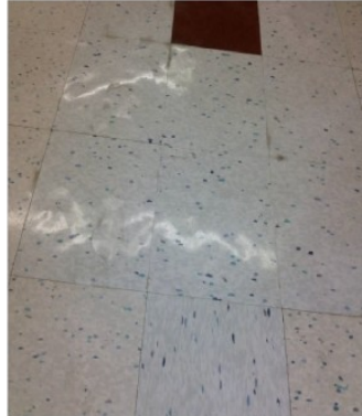
High spots in subfloor getting burned while burnishing Wavy & uneven subfloor telegraphing. Owner did not want to pay for prep, now he's complaining
